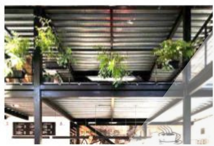
• FINAL VIEW OF MEZZANINE FLOOR DECKING SHEET
