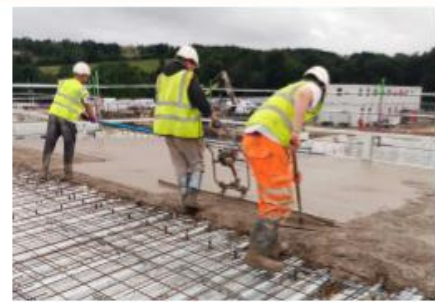
• SETTLING CONCRETE LAYER
